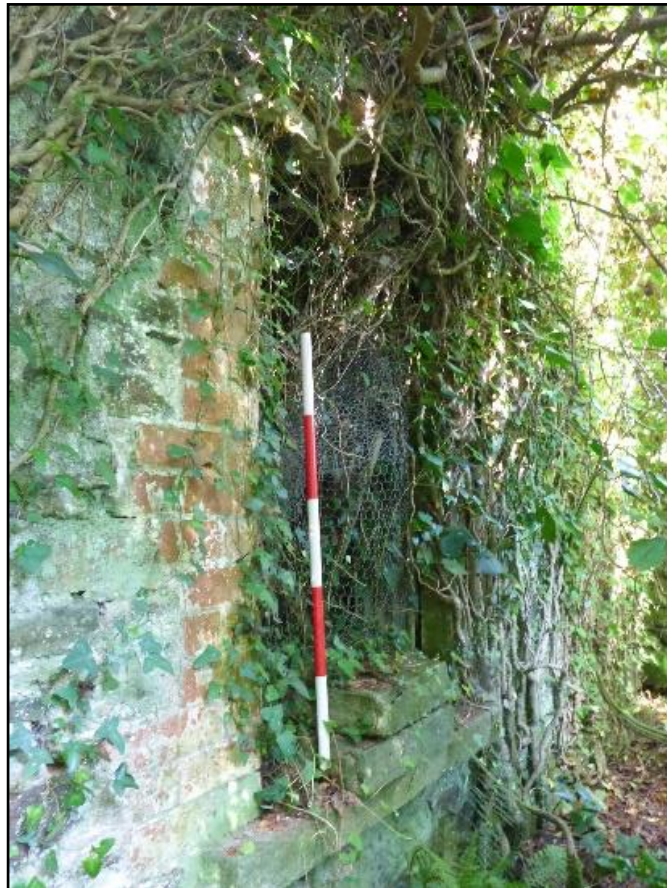
Plate 13-8. Red-brick lined external cottage window.
