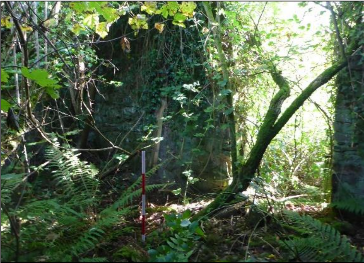
Plate 13-9. Roofless ruin of the outbuilding adjacent to the cottage.
