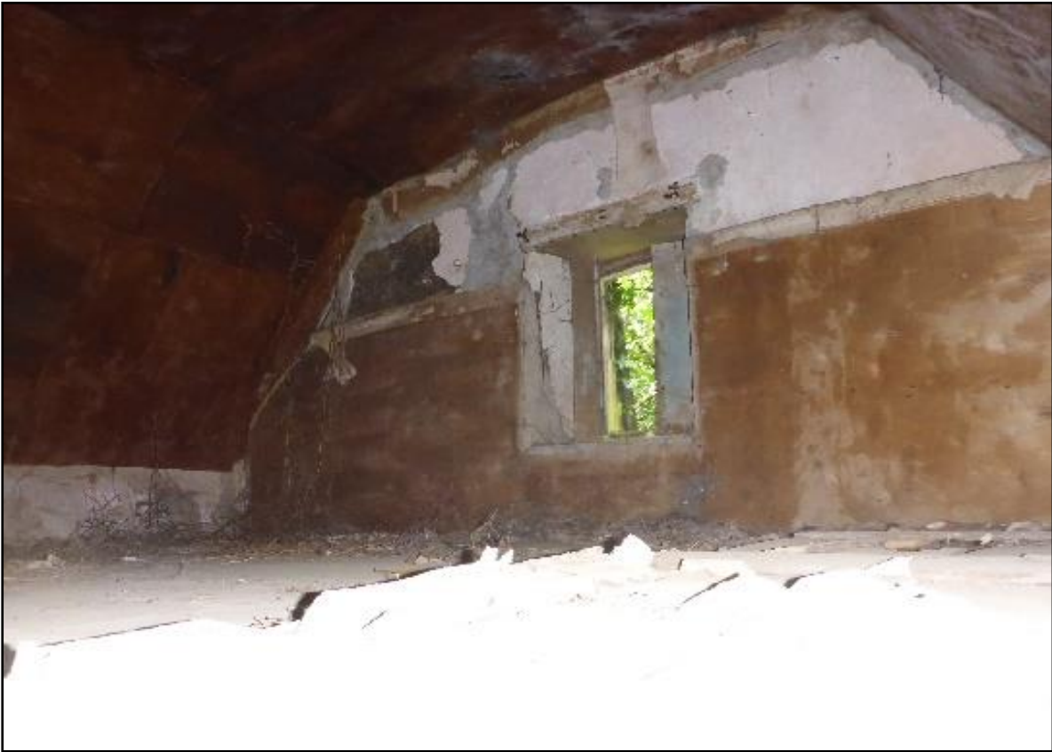
Plate 13-7. Window in north facing gable of loft.
