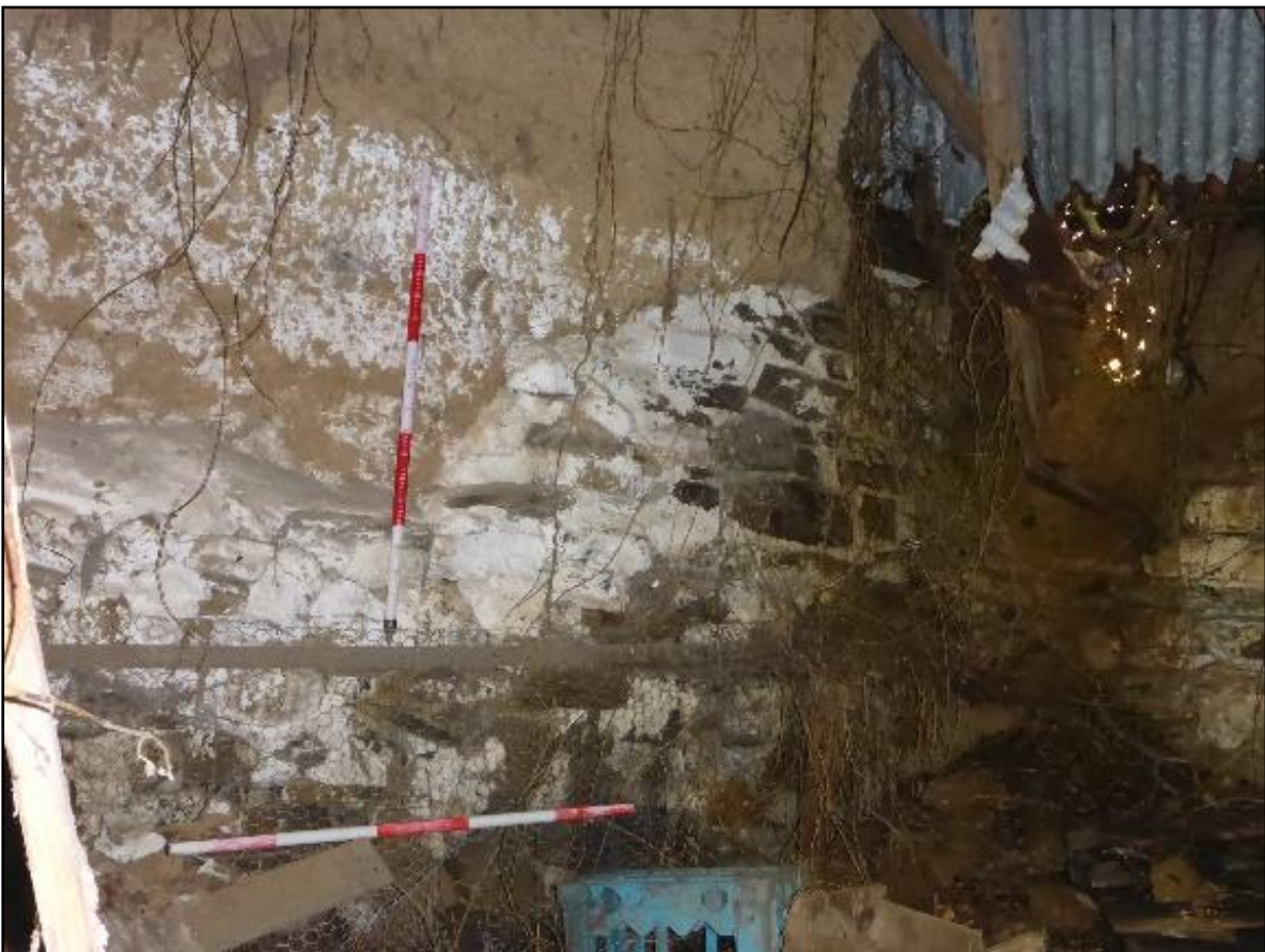
Plate 13-10. Gable end of long barn – stone and mud construction
