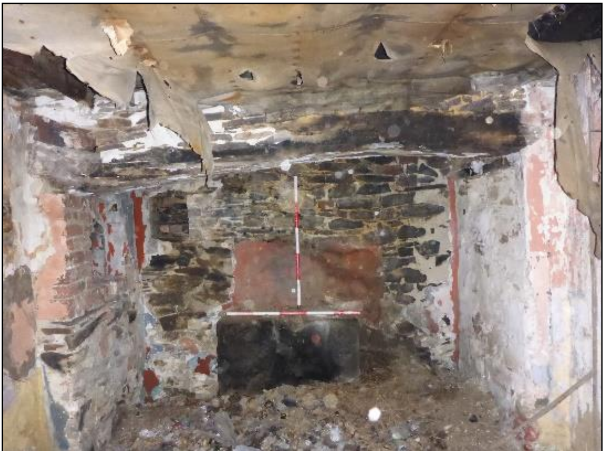
Plate 13-4. Kitchen hearth within cottage (note square keeping hole to the top left)
